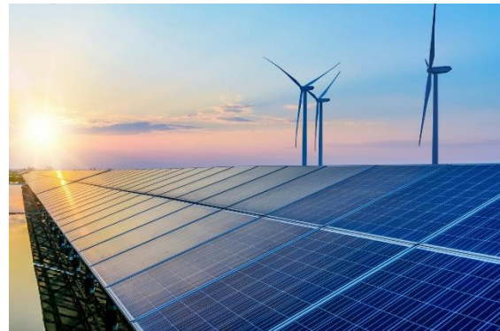
FIG 3: LARGE SCALE SOLAR FARM
