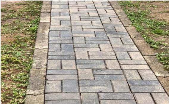
Fig 3.2: plastic tiles used as sidewalks
