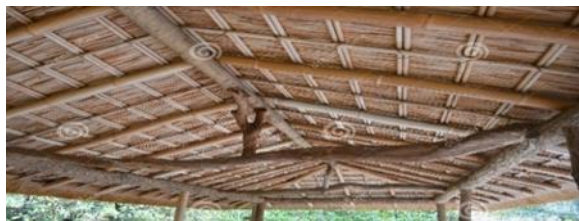
Figure 6- Bamboo Roof Truss
