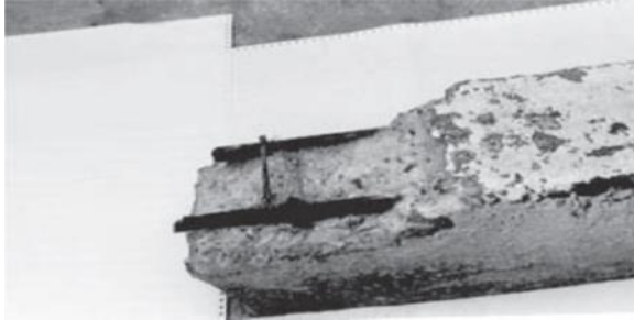
Figure 10 - Bamboo reinforcement after 15 years in open air
