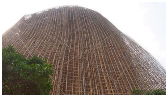
Figure 7 – Bamboo scaffoldings
