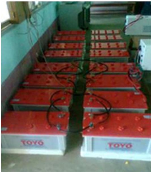
Fig.5. 200Ah batteries for storing the charges for later use
