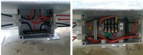
Fig.3 Wire Connection in Connection Box and Fuse Box
