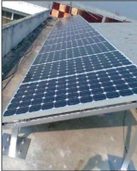
Figure 2. Conversion Efficiency 14%, 16 × 160 W Modules Mounted at the Roof-top of the Class Room
