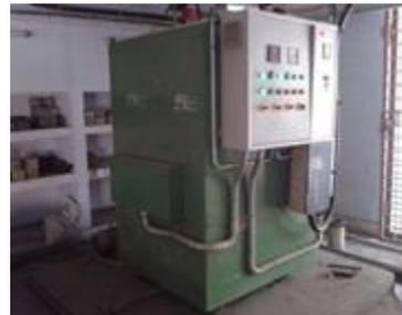
Figure 7 Steam Boiler
