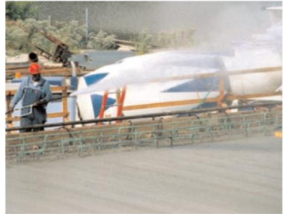
Fig.1 Fogging minimizes moisture loss during and after
