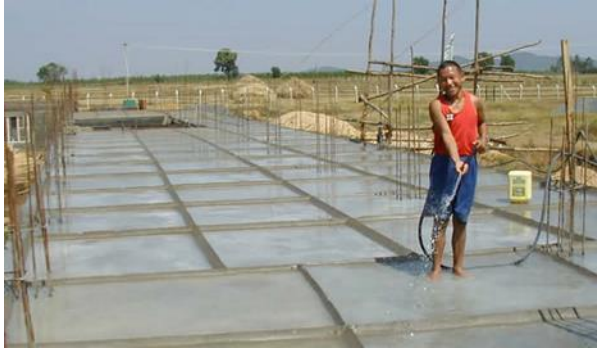
Fig. 2 Ponding method of curing
