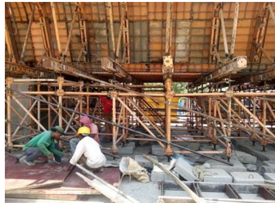
Photo.1. Scaffolding for Bridge Span
