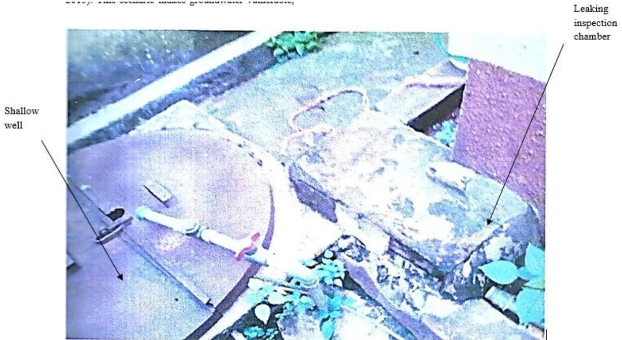
Figure 1: A shallow well with leaky inspection chamber
