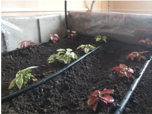
Fig 3(b) - drip irrigation piping system
